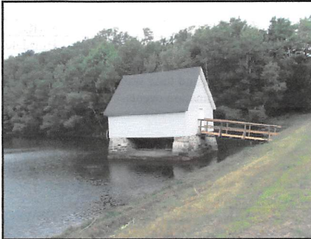
Belmont Reservoir Pump House, Hinsdale, MA.
